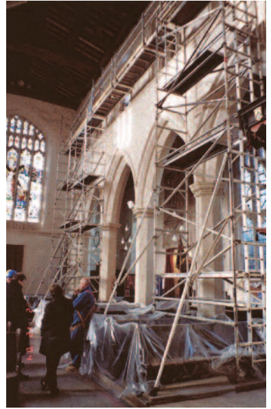
Repairs to clerestory window of St George's Church, Toddington, Bedfordshire.
